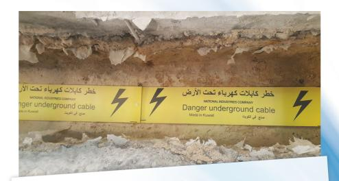
For years, NIC has supplied concrete cable cover tiles to Kuwait market. In view of latest market developments NIC is proud to present NIC HDPE Cable Cover Plates. NIC HDPE cable cover plates are produced by using a latest modern machinery. Unlike concrete tiles, the high density polyethylene (HDPE) plates are extremely tough and do not tend to crack. They comply with impact strength requirement for concrete tiles to BS 2484.
