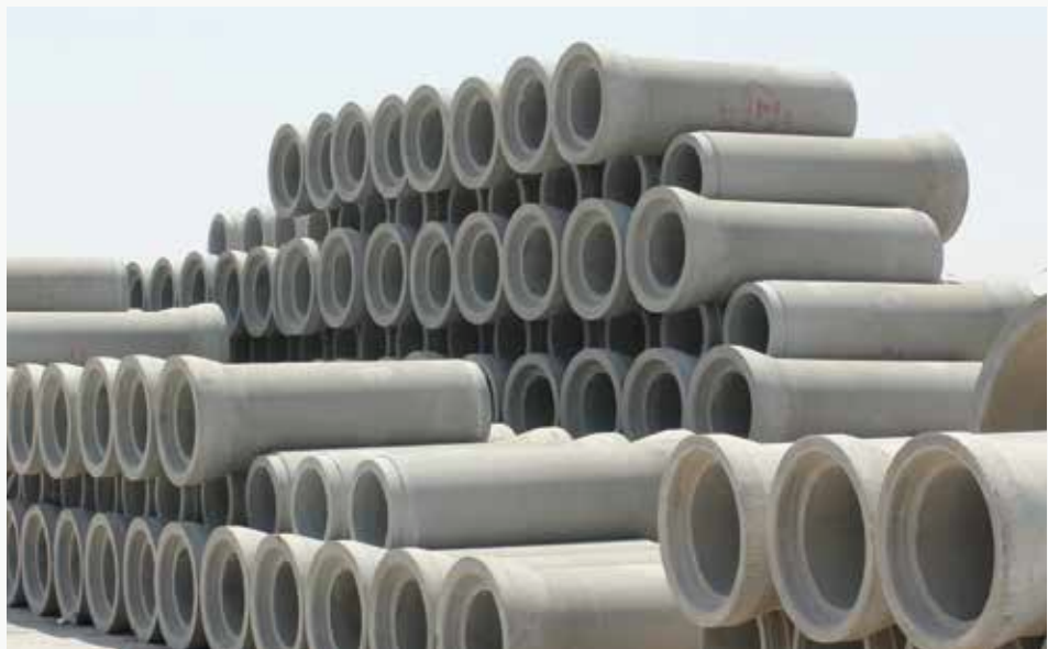
Fig. 2. Shows the correct method for Stacking the pipes.
