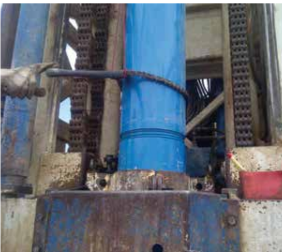
Assembly of Pipes
