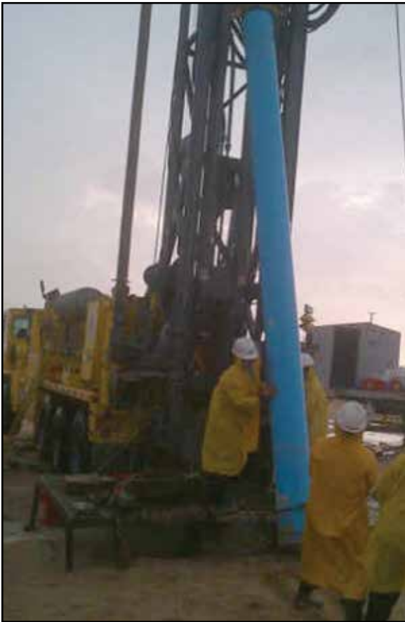
Well Tube Installation
