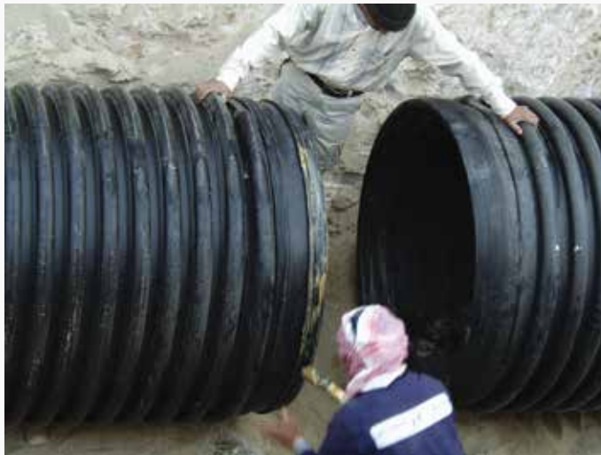
Applying Lubrication to socket and spigot, after cleaning, at Kuwait
