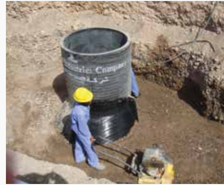
Initial backfill at project in Oman
