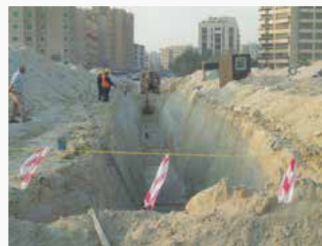
Trenching at Kuwait
