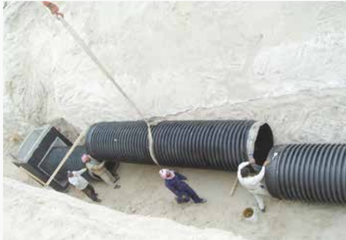
Loading at project in Kuwait
