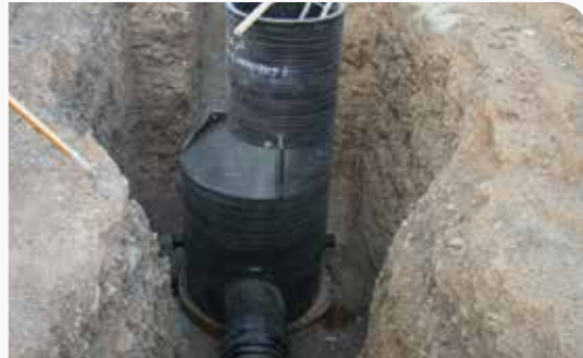
NIC HDPE Corrugated Pipes for Sanitary / Sewerage water, connecting to HDPE Manholes, project in Oman
