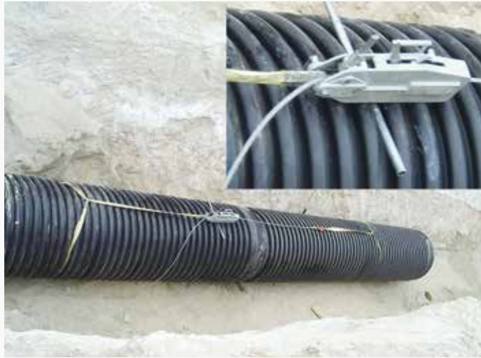
Assembly of pipes at project in Kuwait
