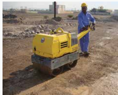
Final Backfill at project in Oman
