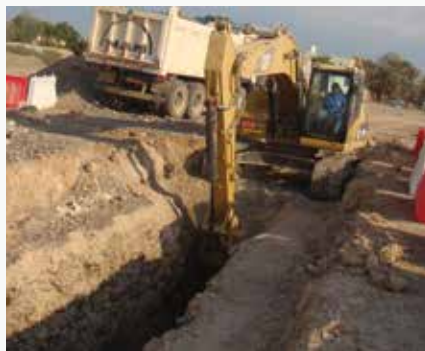
Trenching at Oman
