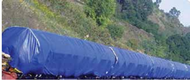
Storage at site
