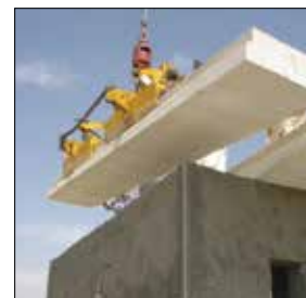
Slab Fixing
